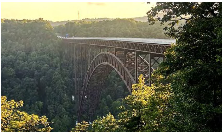
A view of the New River bridge in West Virginia .
