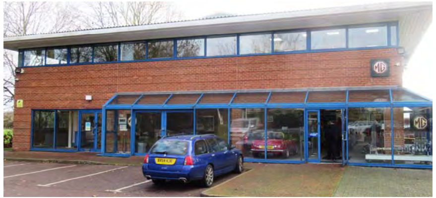
MGOC Headquarters "Octagon House" (actually a rectangle).
