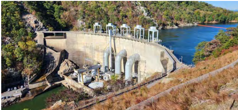
A view of the dam with its power station.
