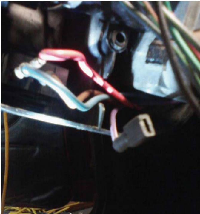
Switch assembly removed
